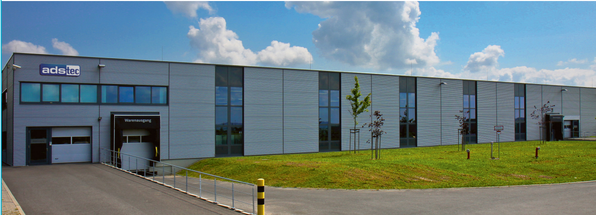
Company headquarters (above) in Nuertingen near Stuttgart, production site in Wilsdruff near Dresden
